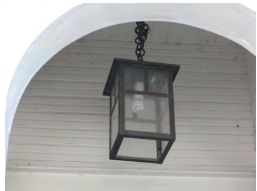
Replacement light fixtures shall be in keeping with the period of the house such as this Craftsman light fixture on a Bungalow style dwelling.
