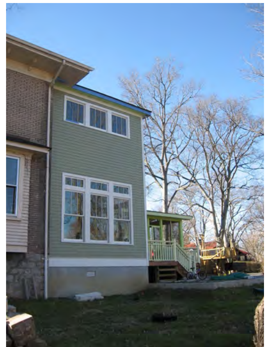
Additions shall be subordinate to the original dwelling and be differentiated through materials and detailing.
