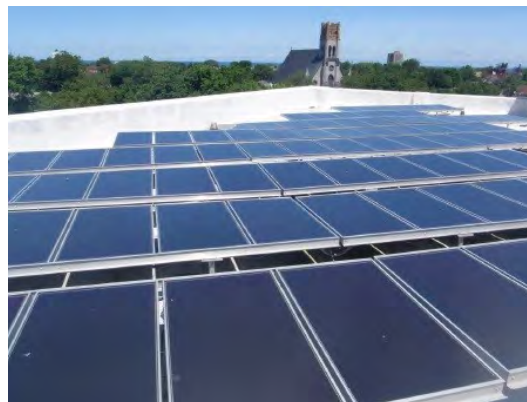
The installation of solar panels on roofs of commercial buildings is appropriate and encouraged. These panels shall be sited below a building's parapet wall and not visible from the street as shown in this example.
