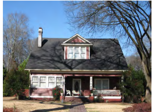
This ca. 1919 Bungalow at 70 College Street displays a recessed porch and a gable dormer at the roofline.
