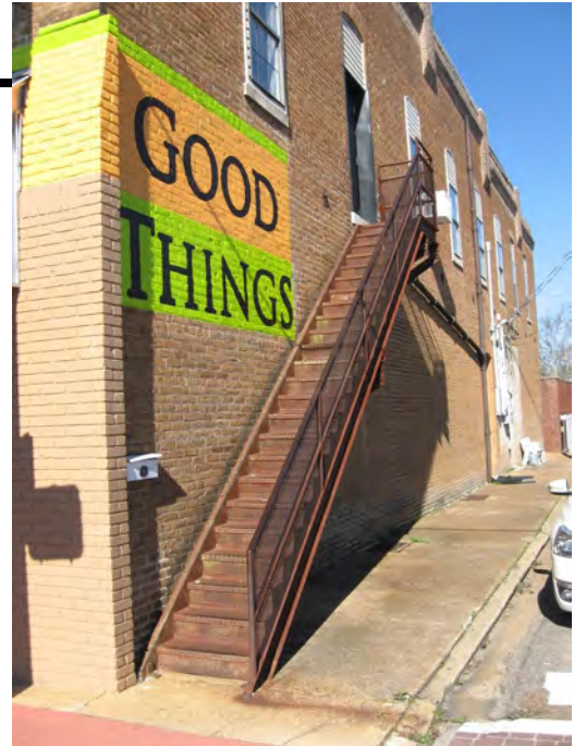
Fire escapes and staircases are appropriately located on side or rear elevations (above, 390 Main Street).
