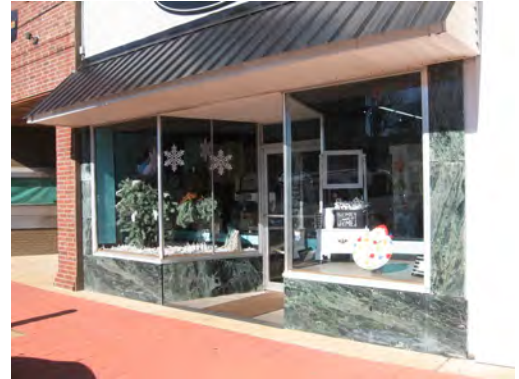
The marble paneled storefront at 430 Main Street (above) and Carrara glass storefront at 407 Main Street (below) are examples of modifications that are now historic in their own right and should be preserved.
