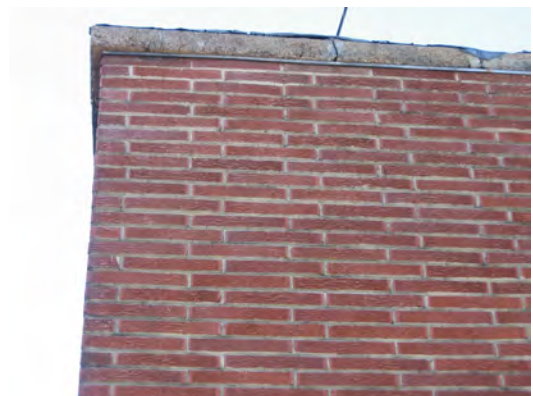
By the mid-20th century, long and thin masonry known as “Roman brick” was used as the exterior surface for some downtown buildings such as at 160-168 Guinn Street.
