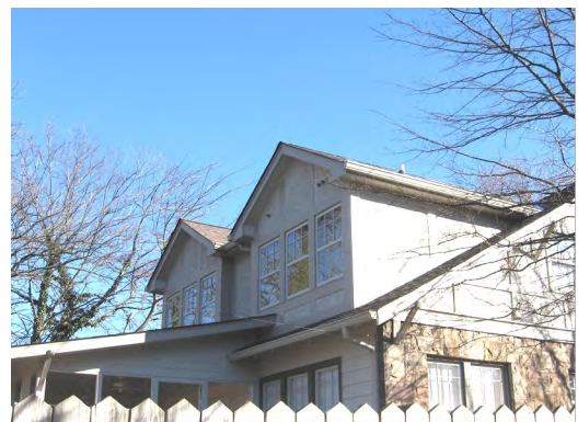
Utilization of unused attics and the addition of rear elevation dormers may also be an appropriate method to add additional living space to a dwelling.
