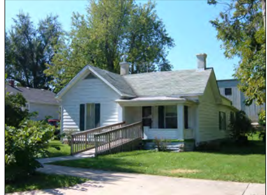
Avoid the construction of a prominent ramp on the front of a dwelling.
