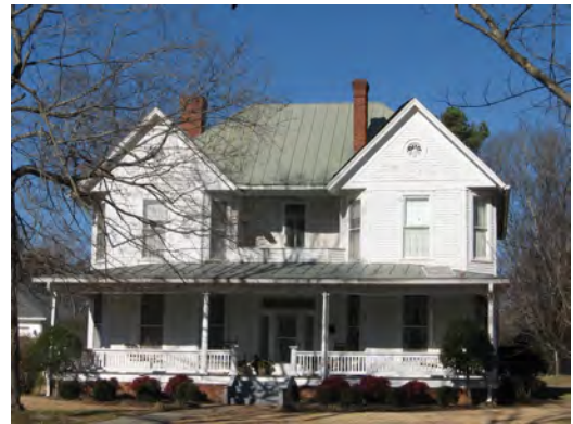
Most dwellings in the Savannah Historic District are of frame construction and reflect popular and vernacular building forms and styles of the late 19th and early 20th centuries (130 College Street).
