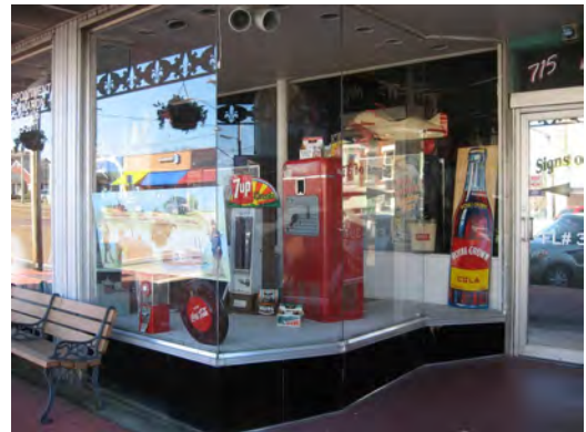
Downtown Savannah contains historic buildings with notable storefronts such as at 385 Main Street. This storefront features black Carrara glass, a tinted glass popular in the 1930s and 1940s.
