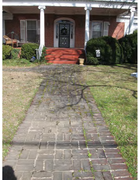
Brick patterns of original sidewalks shall be preserved and maintained (120 Main Street).
