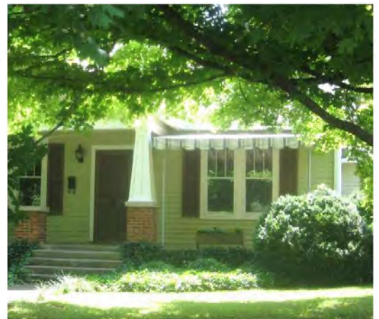
Porches are also appropriate locations for canvas awnings to reduce energy costs in warm months.
