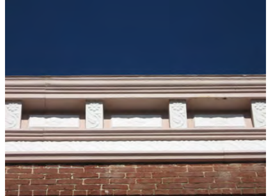
This original sheet metal cornice at 406-408, Main Street is well maintained and is a major feature of this commercial building.
