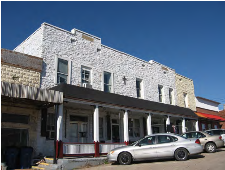
The ca. 1931 building at 250 Guinn Street is constructed of stone veneer, another masonry type within the historic district.
