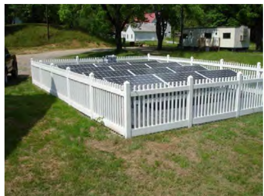
Solar panels may also be added to rear yards as long as they are not readily visible from the primary street and are screened through landscaping or fencing.
