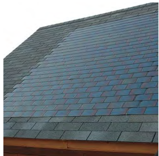
Solar panels (above) and solar shingles (below) may be added to dwellings at their rear roof lines or side roofs not readily visible from the street.
