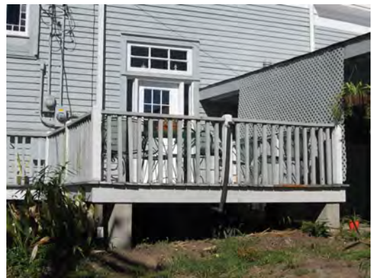
Rear decks shall be built of materials to complement the historic dwelling without removal of original fabric.
