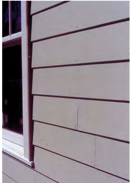
The use of cementitious siding may be appropriate for new construction, repairs on garages and repairs on the rear elevations of dwellings. This kind of alternative siding is not appropriate on elevations of a historic building that are visible from the street.
