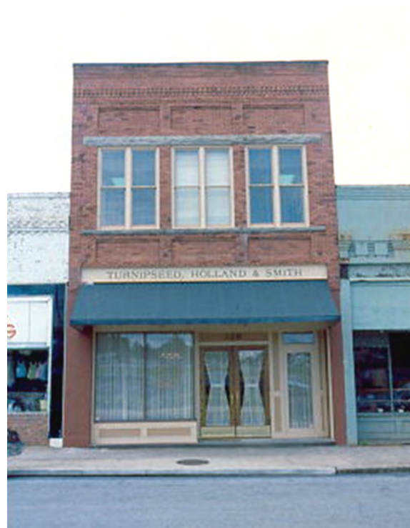
The Secretary of the Interior's Standards recommend preserving and restoring original features. Here the building's storefront and windows were conserved and re-used as part of the overall rehabilitation.
