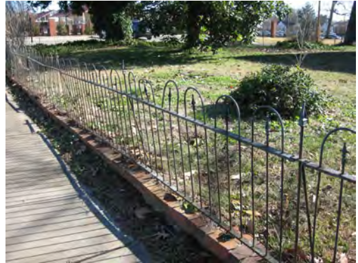
Retain original metal fencing like this hoop and dart fence at 15 College Street
