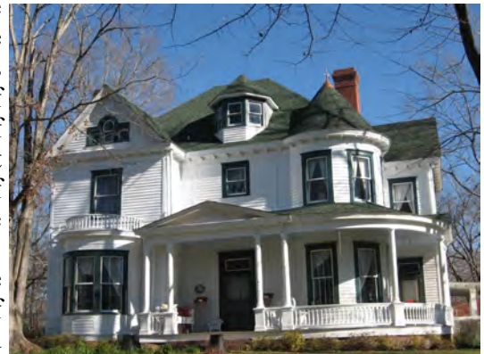
The irregular roof plan and components are character-defining features at the Queen Anne-style dwelling at 200 Church Street.
