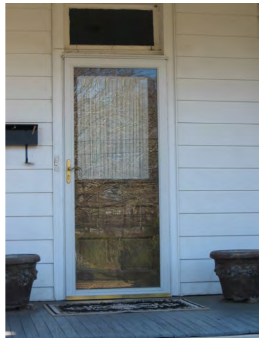
The storm door installed at 215 Church Street is an appropriate design, allowing for full view of the dwelling's original single-light glass and wood door behind it.
