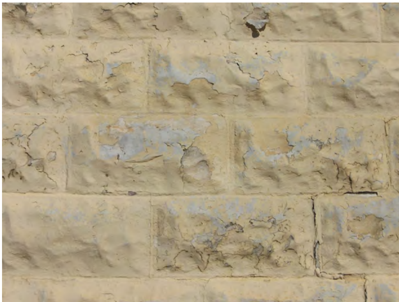
The exterior walls at 470 Water Street are rock-faced concrete block. The guidelines for masonry apply to brick, stone, and block surfaces.
