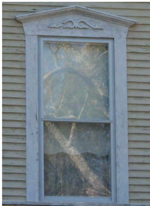
Original one-over-one wood sash window with decorative pedimented surround at 195 Williams Street.
