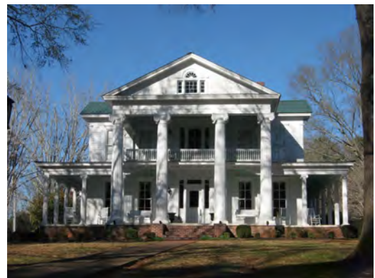
The dwelling at 320 College Street is a notable example of the Neo-Classical style and features a two-story portico with Ionic columns.
