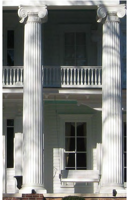
The fluted columns on the portico at 320 College Street feature Ionic capitals.
