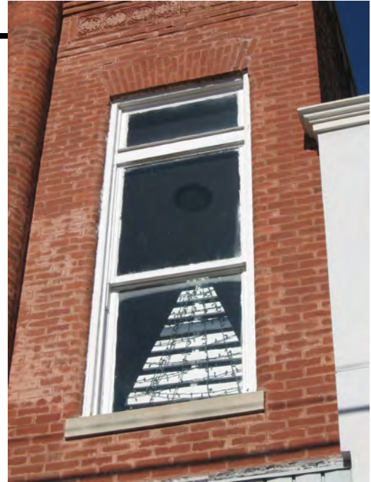
Retain original windows and transoms such as this one-over-one wood sash example at 416 Main Street.
