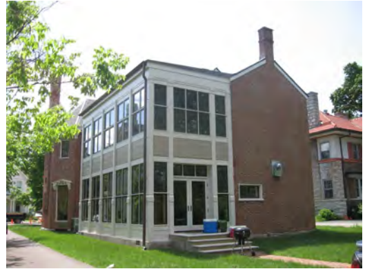
Additions shall be sited at the rear or non-readily visible side elevations.
