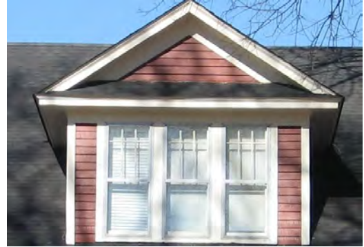
Original six-over-one Craftsman style windows in the gable roof dormer at 70 College Street.
