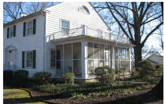
The original screened side porch on the dwelling at 95 College Street is an appropriate example for enclosed porches in the historic district.
