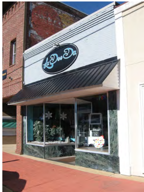
One-Part commercial block building at 430 Main Street.
