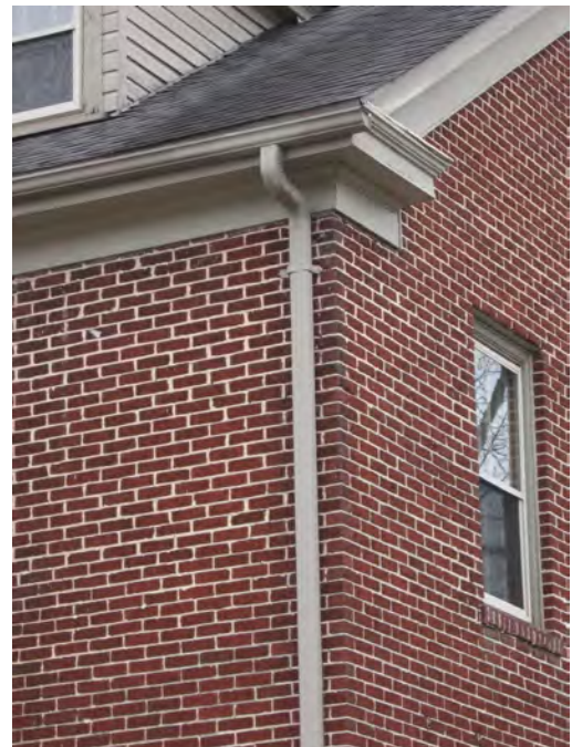
Example of an appropriate gutter and downspout.
