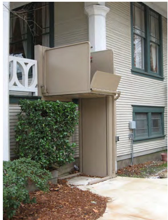
Chair lifts are also a preferred method for accessing historic dwellings. This installation results only in the removal of a small section of porch railing which can be added back when the chair lift is no longer needed.
