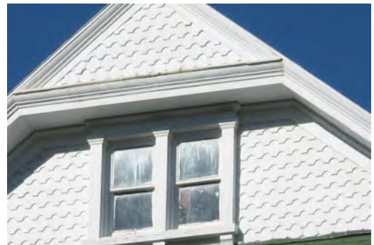
Retain and do not conceal original wood features such as the shingles in the gable field at 155 William Street.
