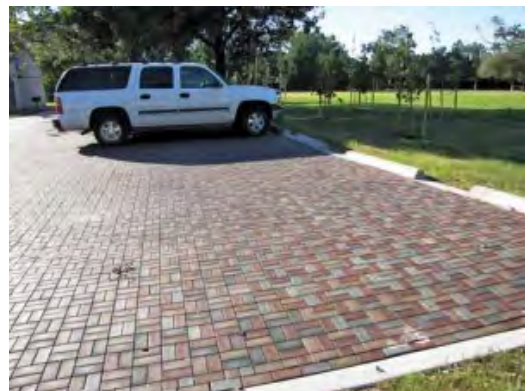
The City of Savannah should consider the use of permeable paving surfaces to allow for absorption of water and less run-off into storm sewers.
