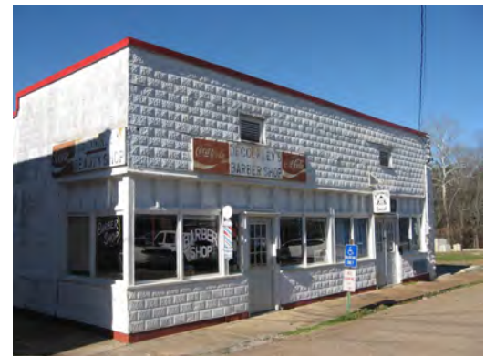
The exterior walls at 585 Cherry Street are covered with pressed tin panels that mimic rock-faced concrete block.
