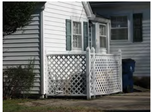
This HVAC unit is effectively screened through lattice panels at 165 College Street.
