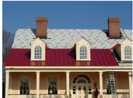
New metal roofs shall match historic profiles of crimping and spacing to match original metal roof designs of the dwelling's period.
