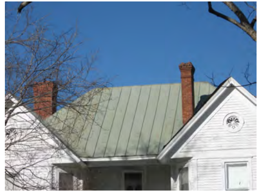
The dwelling at 130 College Street retains its original metal standing seam roof—these types of roofs should be repaired and retained.
