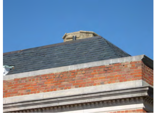
Preserve distinctive roof features and materials, such as the slate roof at the Tennessee River Museum (above) and the pressed metal shingles on the tower of 416 Main Street (below).
