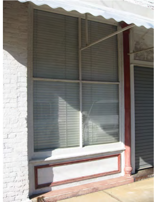
This original storefront at 242 Guinn Street retains its frame bulkhead, four-light display window, transom and cast iron column.
