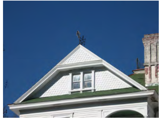
Exterior wood siding requires thorough scraping and priming prior to painting (155 Williams Street).
