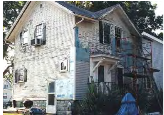
The application of vinyl siding often involves the removal of original historic features and can cause condensation in the walls.
