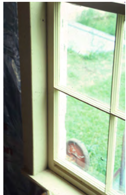
If replacement windows are necessary they shall have divided lights as shown above rather than applied muntin bars.
