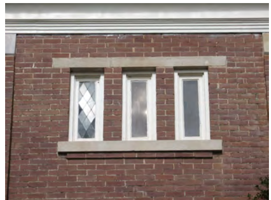
Unpainted masonry walls shall be left unpainted unless the brick is badly damaged or has numerous repairs (First Presbyterian Church, 300 Tennessee Street).
