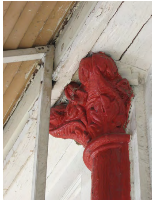
Cast iron was a popular feature on commercial buildings of the late 19th century, as seen at 242 Guinn Street. This cast iron was produced by the Mesker Company of St. Louis and there may be other cast iron features hidden beneath added storefront materials in the downtown area.
